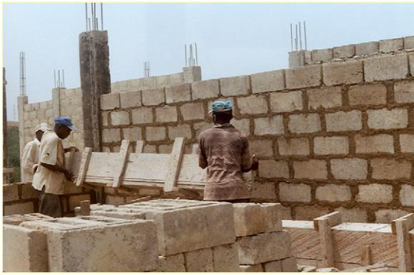
Fig. 4. Concrete blocks and mortar as the major building materials for LRBT.
