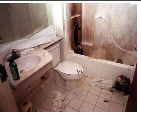
The production process can severely impact surfaces and fixtures.
